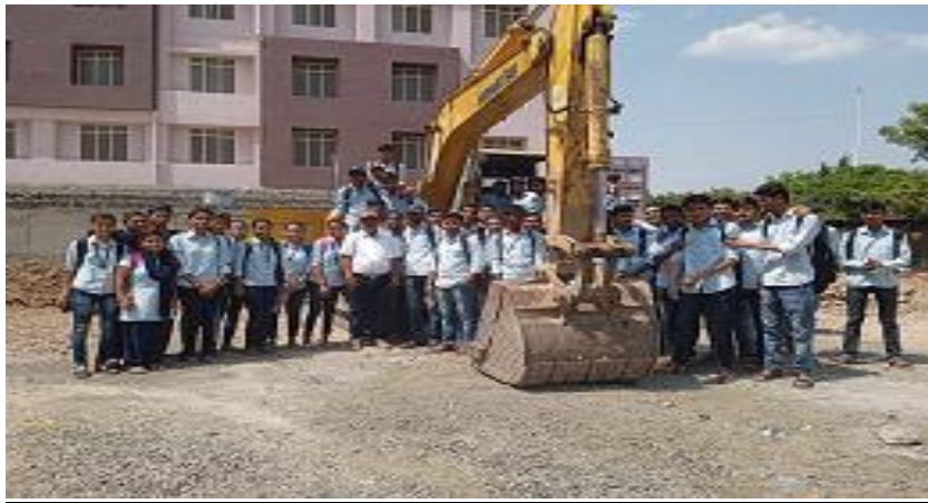
Construction Site At P L G P Latur
